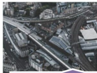
$115bn to modernise bridges and roads
